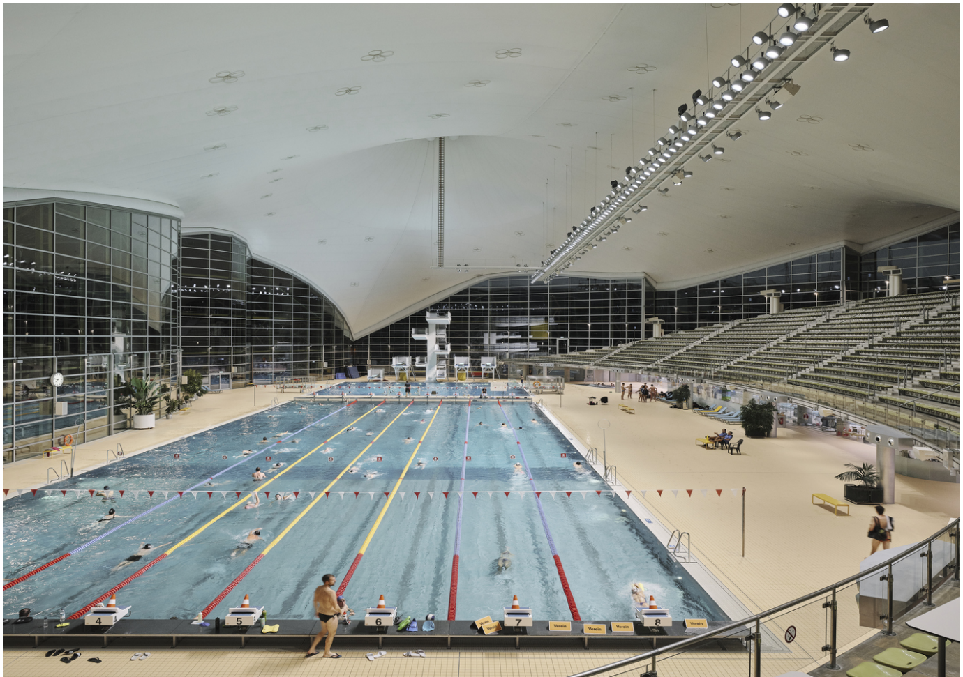
Aquatic Centre at Olympic Park, Munich. Cli- ent: Stadtwerke München GmbH. Architecture: Behnisch & Partner (archi- tect), Otto Frei (roof construc- tion), Stuttgart / Planplus GmbH Architek- ten, Munich (remodelling, refurbishment, project plan- ning). Electrical engineering: Ingenieurbüro Riemhofer, Munich, Paul and Michael Riem- hofer, Munich. Lighting design: 3lpi lichtplaner + beratende ingenieure partnerschafts- gesellschaft mbh, Munich, Beatrice Seidt, Florian Zach. Construction management: ap architektur und projekte gmbh, Munich. Photo- graphy: David Schreyer.
