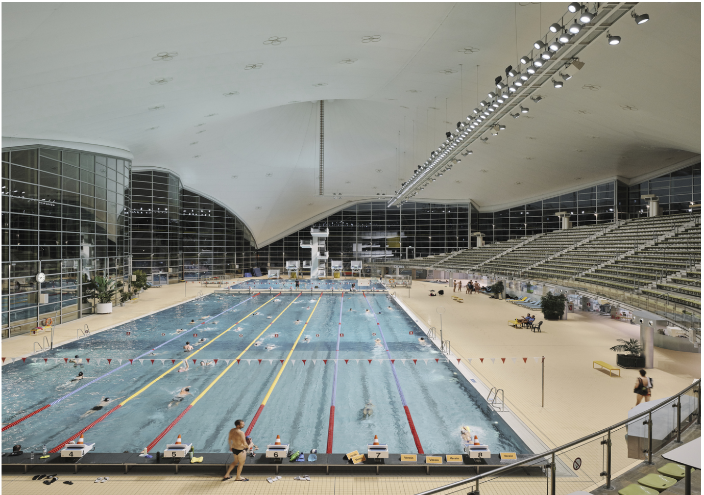
Aquatic Center at Olympic Park, Munich. Client: Stadtwerke München GmbH. Architecture: Behnisch & Partner (architect), Otto Frei (roof construction), Stuttgart / Planplus GmbH Architekten, Munich (remodeling, refurbishment, project planning). Electrical engineering: Ingenieurbüro Riemhofer, Munich, Paul and Michael Riemhofer, Munich. Lighting design: 3lpi lichtplaner + beratende ingenieure partnerschaftsgesellschaft mbh, Munich, Beatrice Seidt, Florian Zach. Construction management: ap architektur und projekte gmbh, Munich. Photography: David Schreyer.
